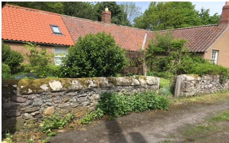
Figure 31: Pantile roofs
